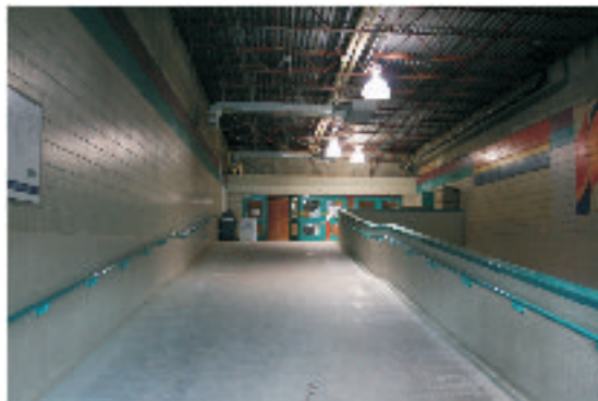
East side ramp view from doors
