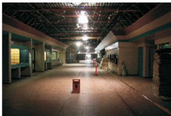
Upper Concourse ceiling is removed
